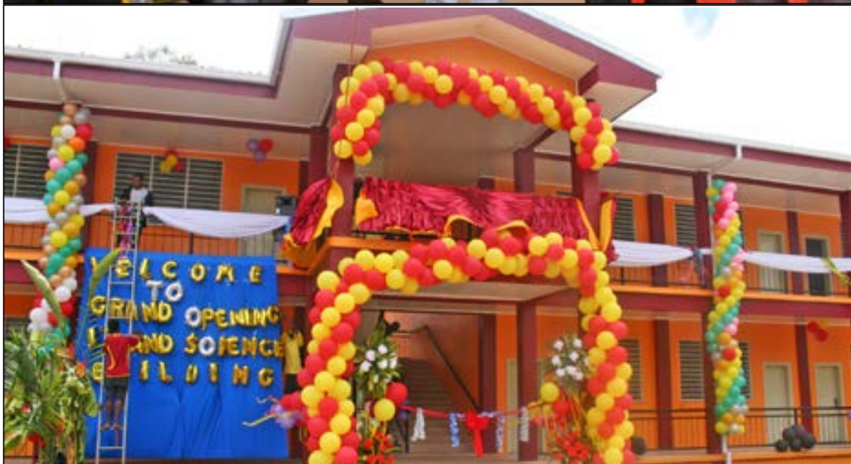
Official opening of double classroom in 2019 by Minister for Education Hon. Joseph Yopyyopy, MP. The classroom was constructed by Pantreid.
