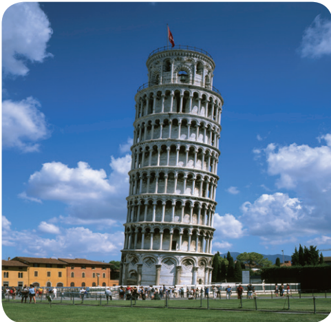
(B) The Leaning Tower of Pisa in Italy: It has a lean of 5^\circ towards the south.
